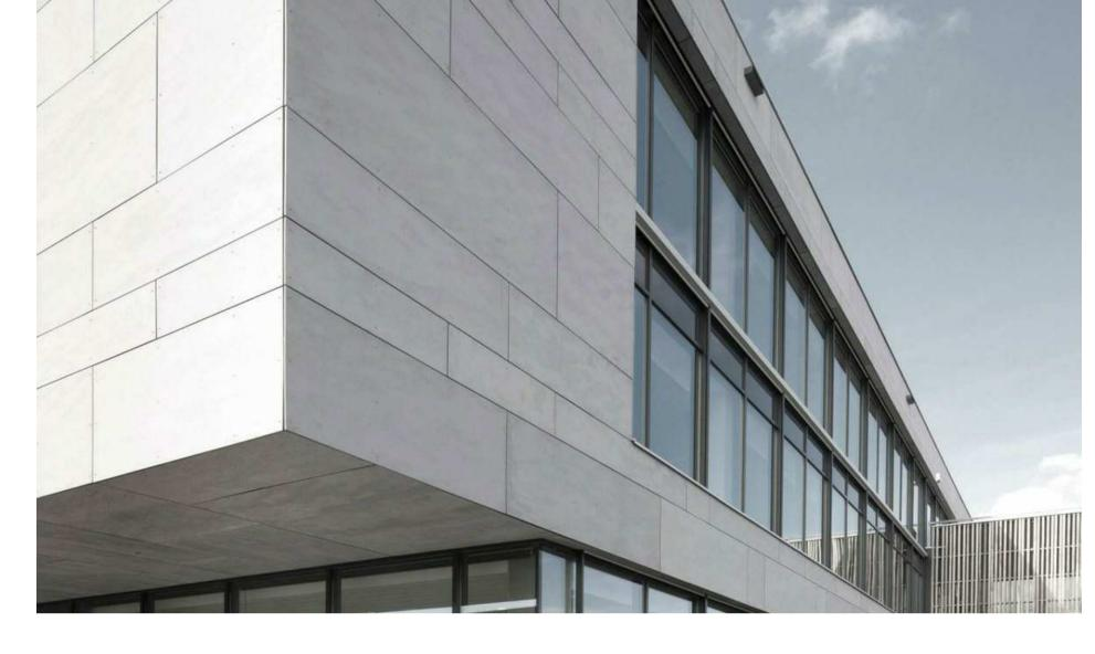
PANELISED CLADDING TO ENDS AND STRUCTURAL SUPPORTS - EQUITONE OR SIMILAR
